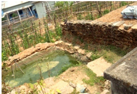
Figure 6a. Waste water from drinking water tap collected in plastic-lined pond to feed plants next to the pond
