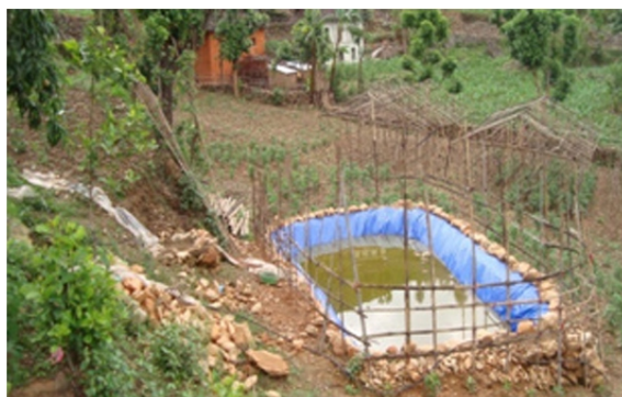
Figure 6b. Silpaulin-lined water harvesting pond that accumulates runoff water channeled via a plastic-lined canal
