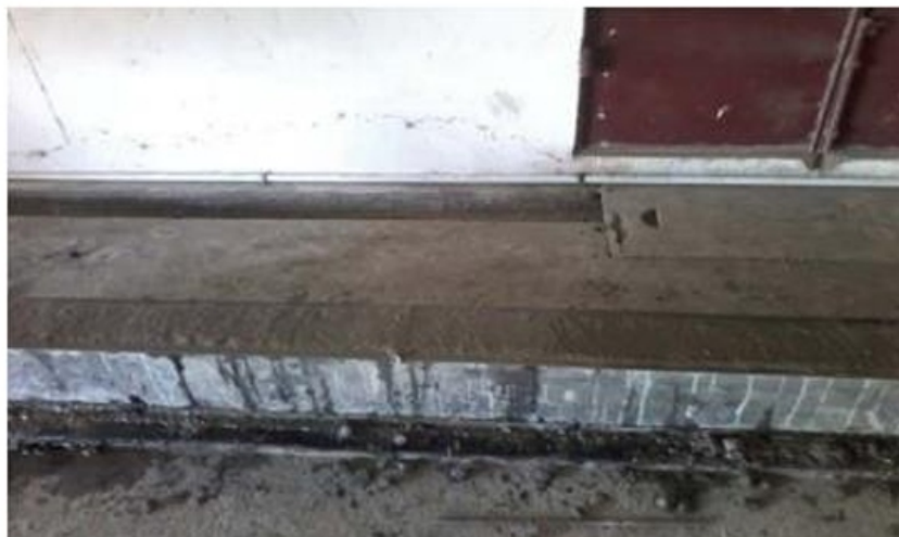
Fig 2 Casting of Beam and surface finishing
