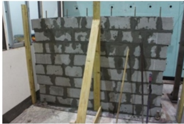
Figure 4. Completed interlocking block wall section with rebar
