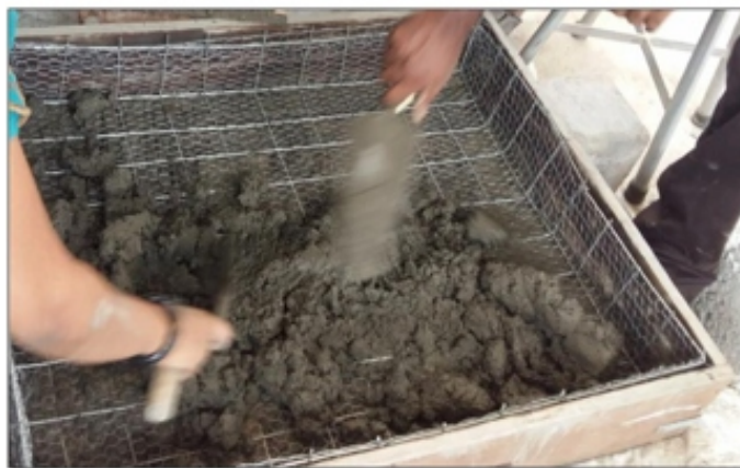
4 Experimental set up of wall panel
