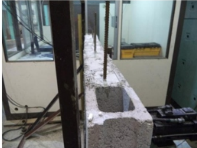
Figure 2. Regular concrete test wall under construction
