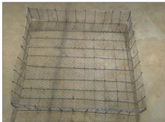
Figure.2 Reinforcement cage with GI wire and wire mesh
