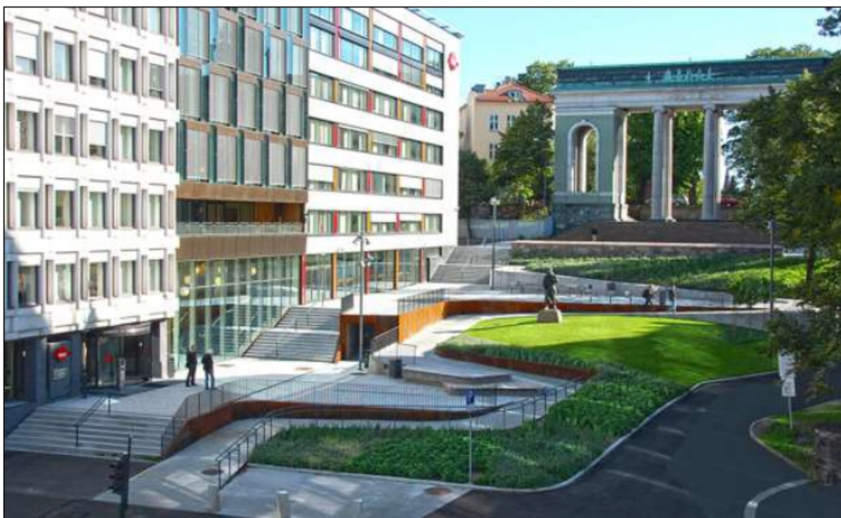
Figure 2. Schandorff Square view [6].
