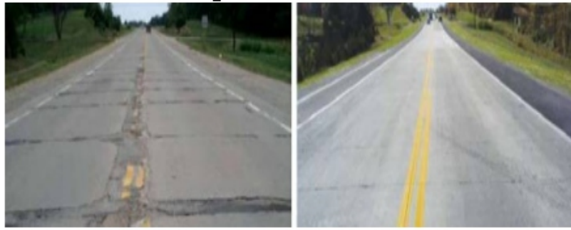
Figure 1: Typical concrete overlay (before [left] and after concrete overlay placement [right])
