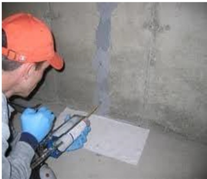
Figure 2: Repair of cracks by Epoxy-injection method [24]
