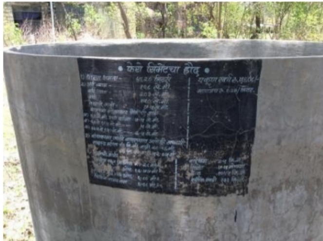
Water tank built in MERI Nashik in 1988
