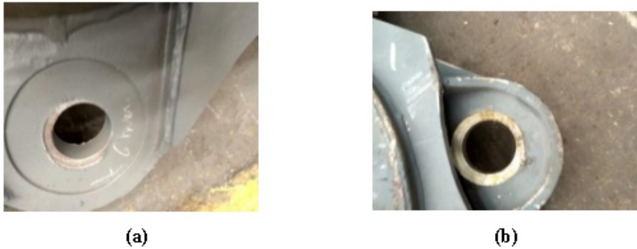
Fig.6 (a)Improper level of bolster guide hole and (b) rectified guide hole after machining and boring This error can be rectified by heating the unlevelled surface, and now machining can be done properly. There are 4 guide holes on the bolster
